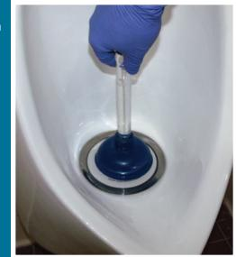
If cartridge flow is slow, extend the cartridge life by: removing the dome; pouring water into the bowl; use a plunger to increase the flow; pour water into the cartridge; and replace the dome. The cartridge should be replaced soon after using the plunger.
