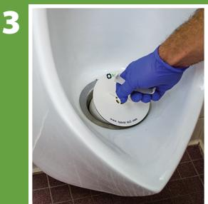
Carefully move side-to-side while applying upward pressure. Lift & remove cartridge. Properly dispose or recycle cartridge. Save tool for future use.
