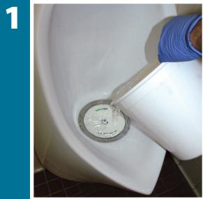
Pour water into the cartridge during routine cleaning. Dome removal is recommended for this "flushing" of the system.
