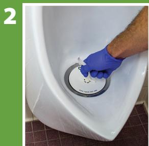
Twist removal tool clockwise onto center stem of the cartridge until snug. Do not over-tighten.
