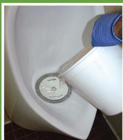
Insert new cartridge and fill with water.
